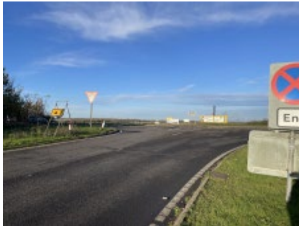
Photograph 2 - (OS Grid Ref: TL 17187 61297)
